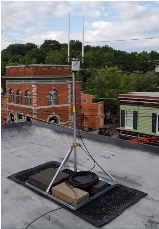
Figure 2 Non-penetrating roof mount (EZ-NP-60-200)
